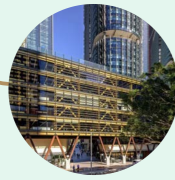
2018 International House Sydney Australia's first engineered timber commercial office building
